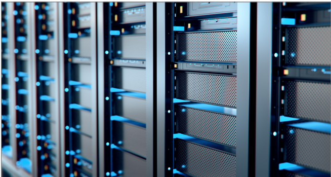
Setup for continuous automated testing
